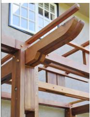
Installation was the biggest challenge in this unique pergola project. While it is actually quite massive, it seems to float off the back of the house and the assymetrical posts line up beautifully. This was accomplished with steel beams attached to the front posts while have enough strength to hold up the entire structure. The view from above adds interest from the second story of the house.
